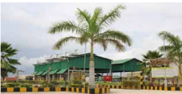
Kigamboni Pump Station, Kilometre Zero (Km 0) this is where It starts from.
